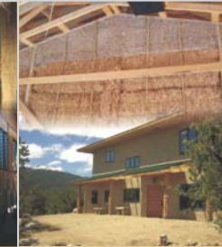
Straw Bales Straw bales provide an extremely strong building block for homes.
