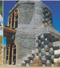
Earthships To build an earthship, you fill old car tires with earth and stack them like bricks.
