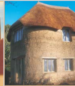
Cob Cob is a combination of earth and straw that you usually mix with your feet, and then form into lumps that you mash together by hand to form the wall.
