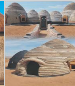
Earthbags Earthbag homes, are made of polypropylene or burlap bags stuffed with dirt and stacked like bricks.
