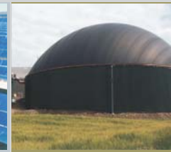
Bio gas Plant - Consumption of organic waste: This biogas technology uses high calorie feedstock consisting of starchy or sugary materials.
