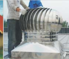
Wind turbine ventilators: Wind turbine ventilators are exactly as the name implies, they are a ventilator that is powered by the wind to create effective ventilation for different industries.
