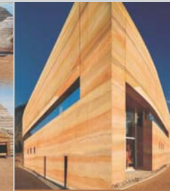
Rammed Earth To build a rammed earth home, a mixture of soils is packed down into a temporary wall form that shapes the mixture.
